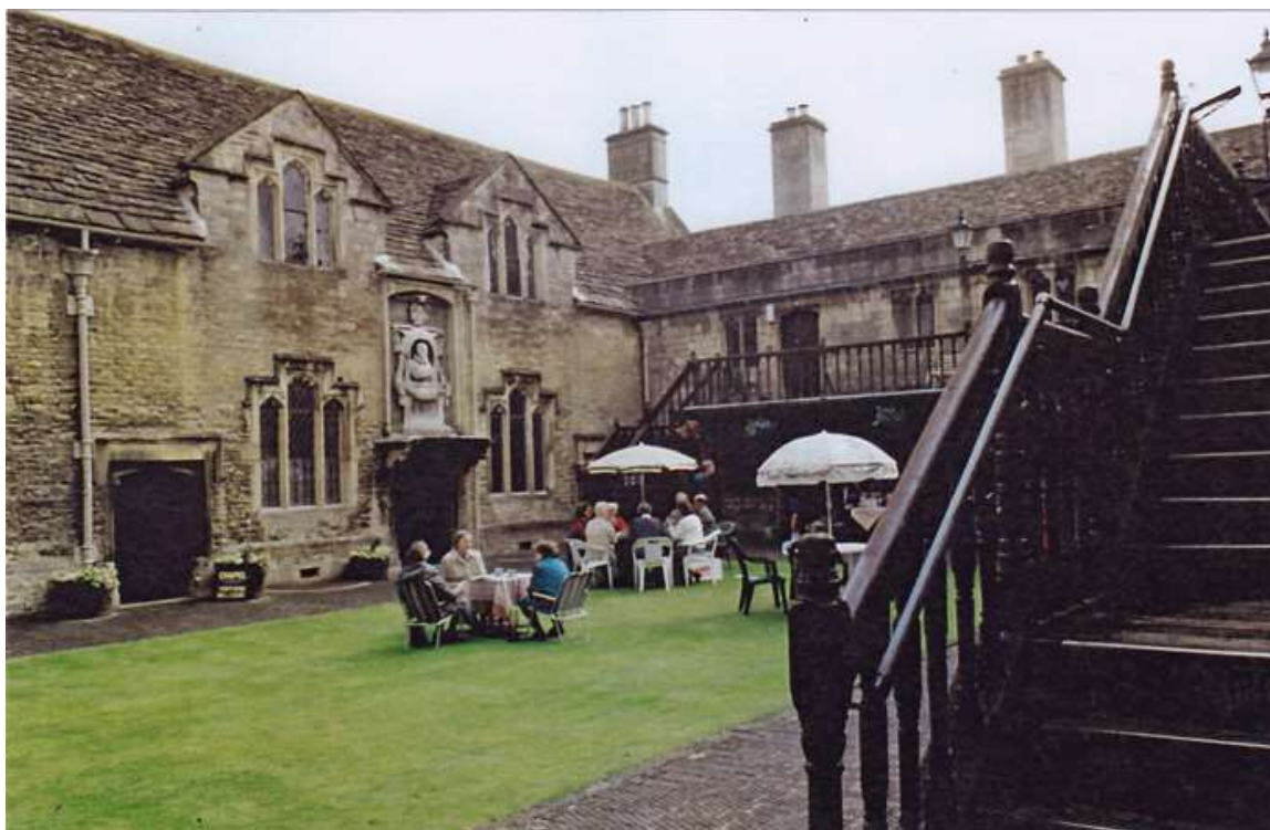
Open Day at Bruton Hospital, 1998. Photo: Mike Chapman.
